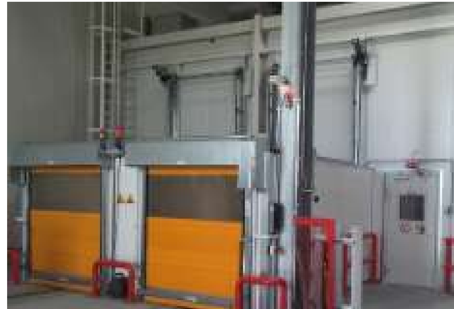
Side view with two airlocks for importing small parts, equipped with two roller doors (at the rear) and two doors automatic sectionals (front)
