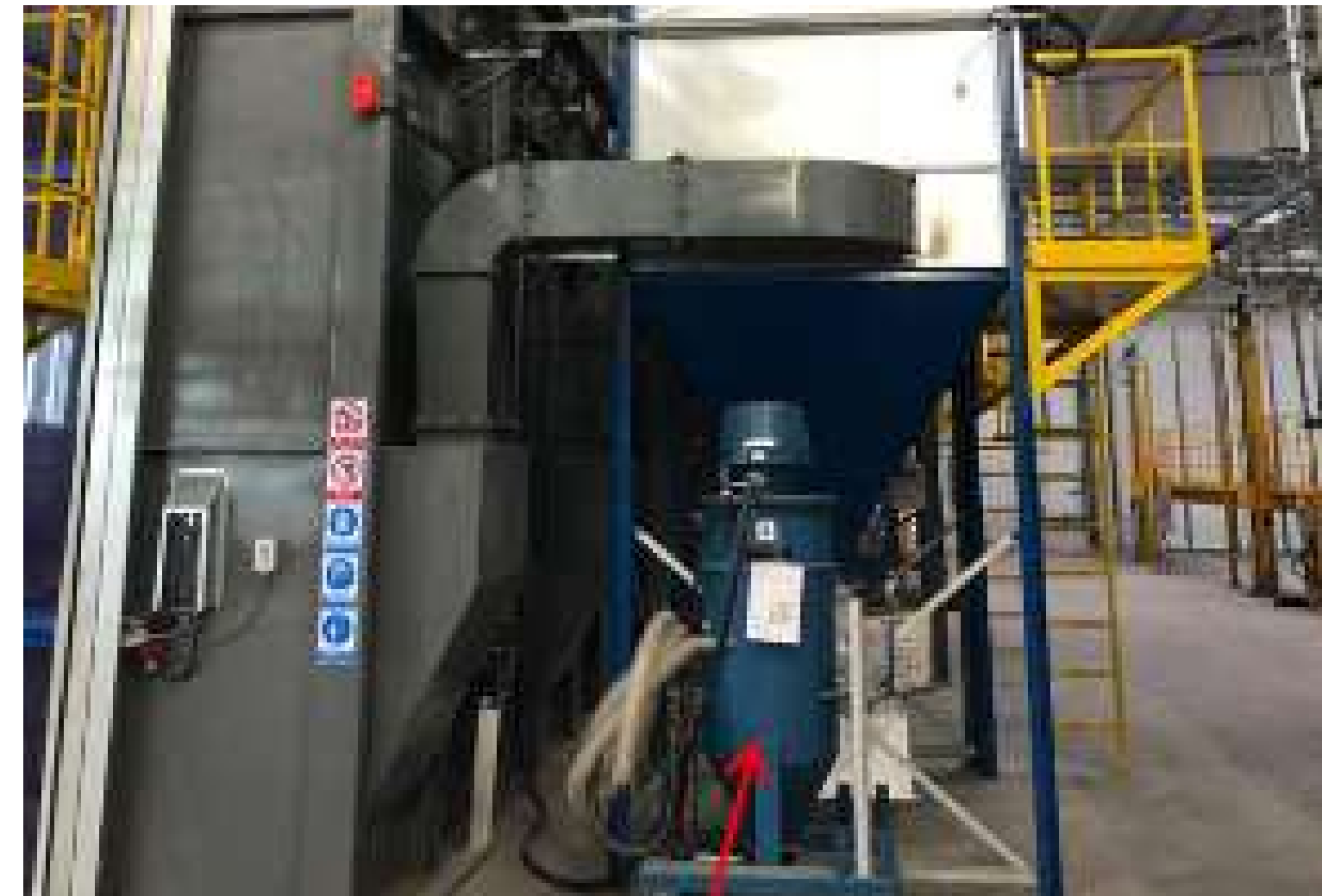
Mobile abrasive resuction installation
