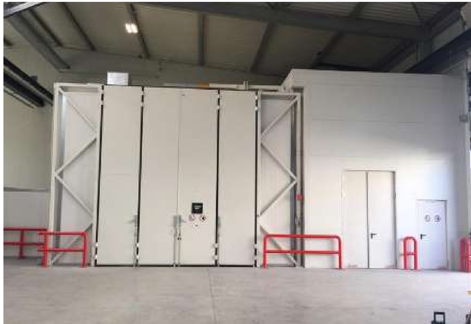
Front view of sandblasting room with hanging folding front door for loading large parts
