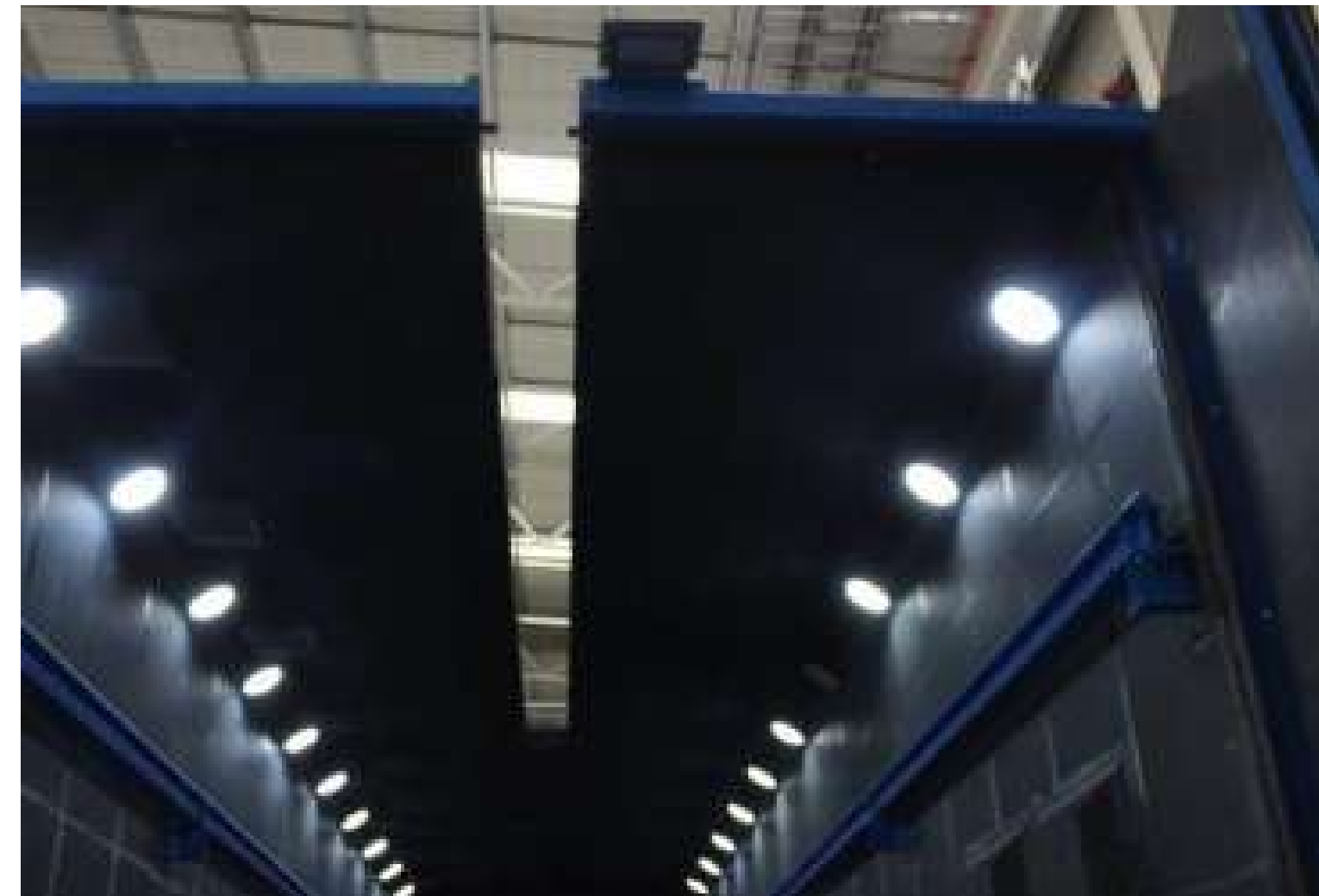
Ceiling slot 11 x 0.5 m, with powered ceiling flap, enables the use of a bridge crane.
