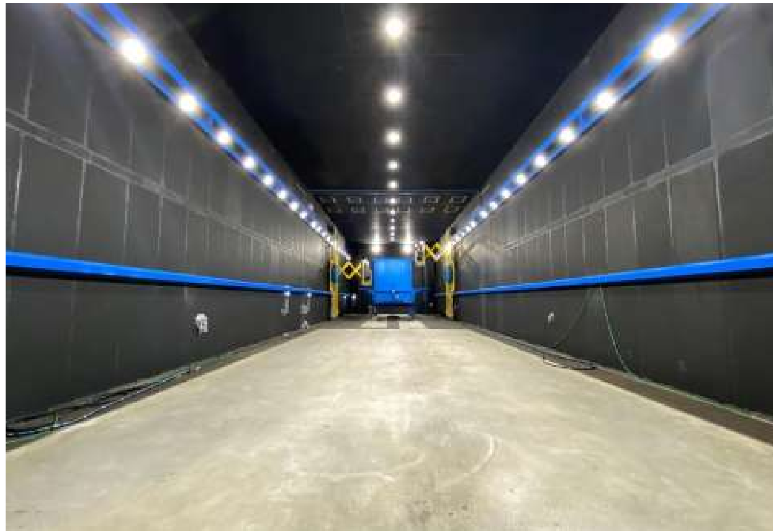
Interior view of a sandblasting room
